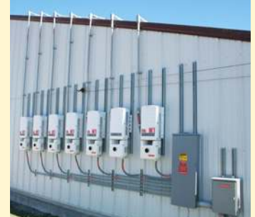
▲ A set of string inverters
