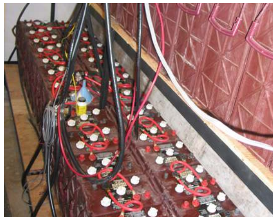
▲ A battery bank
