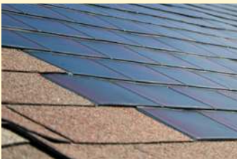
Amorphous thin film solar cells
