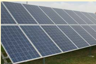
Multicrystalline or polycrystalline solar cells
